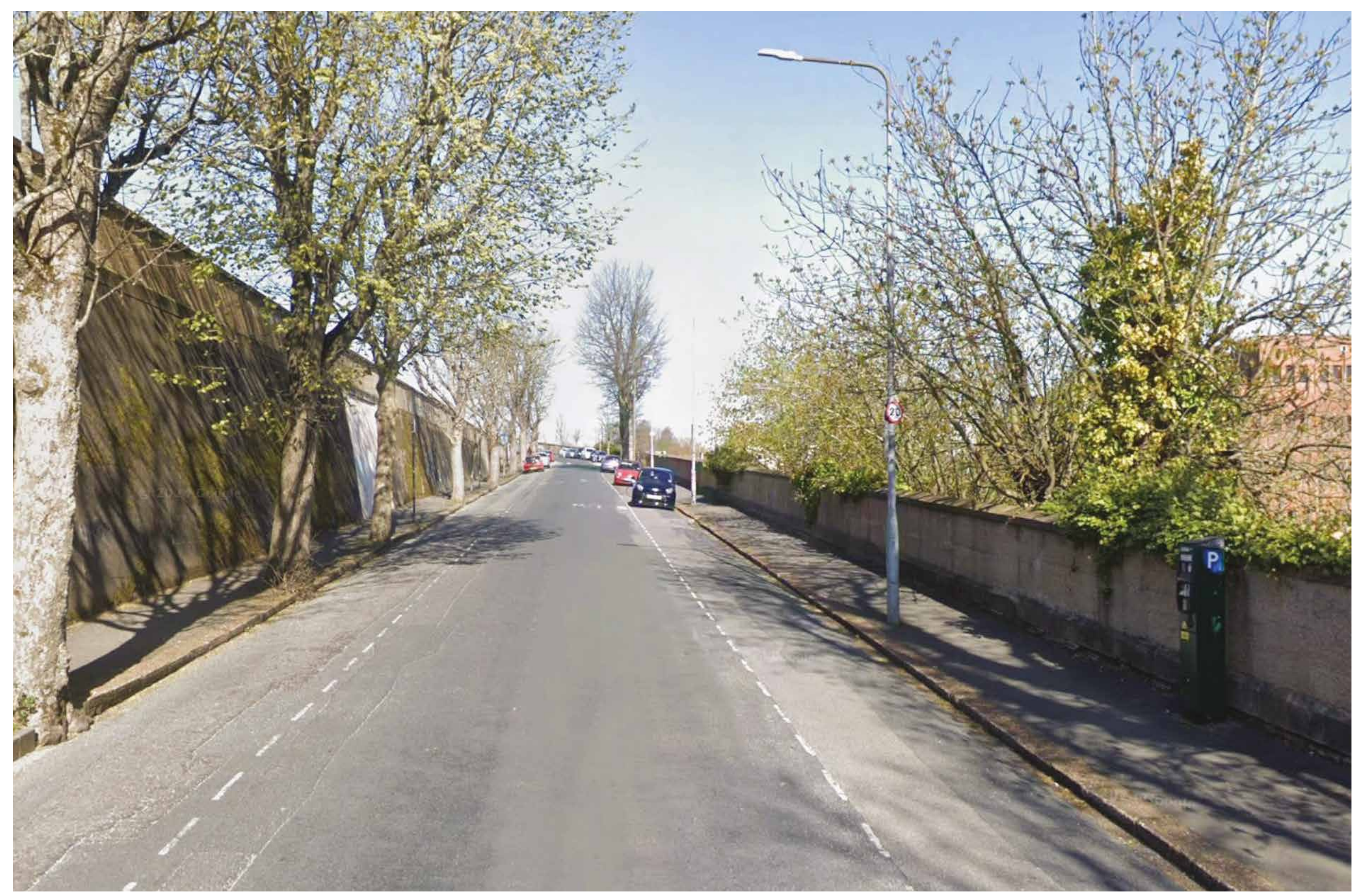
View from Dyke Road Drive showing the change in levels from the mainline railway line (on the left) and the site (on the right)
